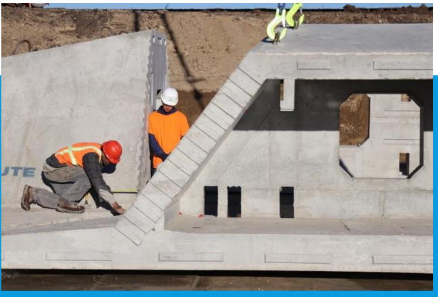
MANUFACTURED FOUNDATIONS FOR WIND TOWERS
